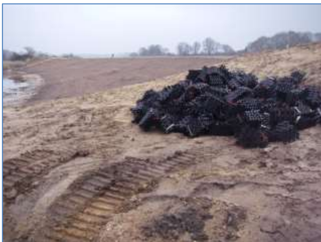
Cellular HDPE mats (Tenax) delivered on site
