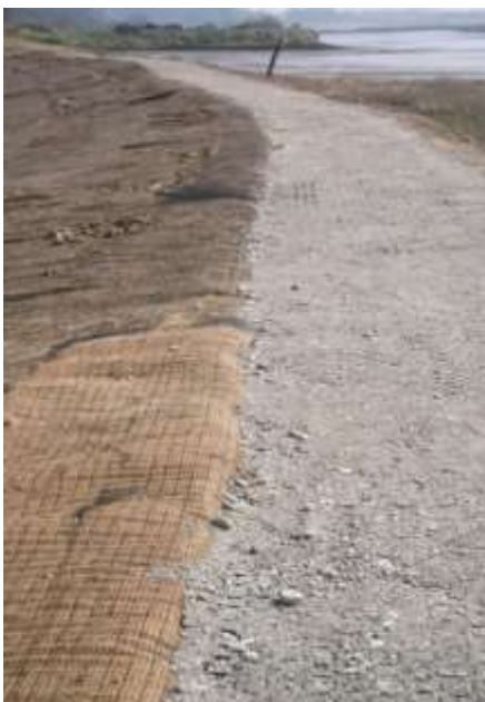
Finished path (looking east)
