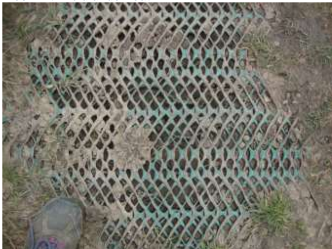
Mesh with void underneath
