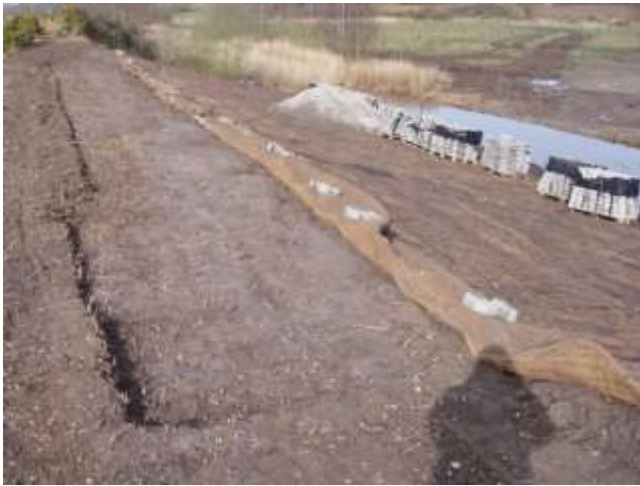
Site strip prior to mesh placement (looking west)
