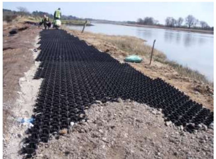
Partially complete of path surfacing across western spillway (looking east)
