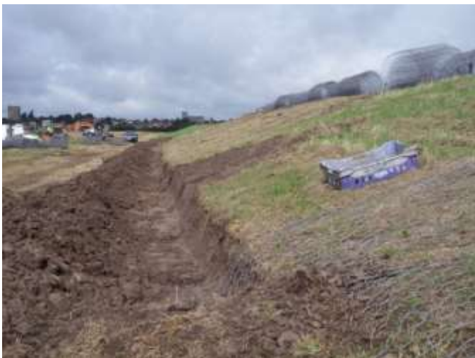
Example of the double twist rockfall mesh used on the wall as the foundation for the interlocking Ankalok blocks. This illustration is from a previous defence repair at Orford.
