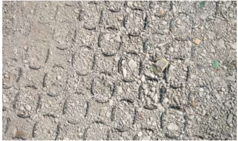
Close up of finished surfacing
