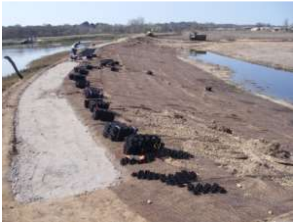
Foundations prior to mat placement (looking west)
