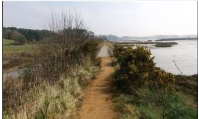
Existing hoggin path looking east towards spillway 2
